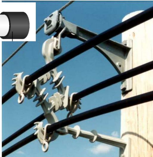
Line with covered cable SPACER CABLE.
